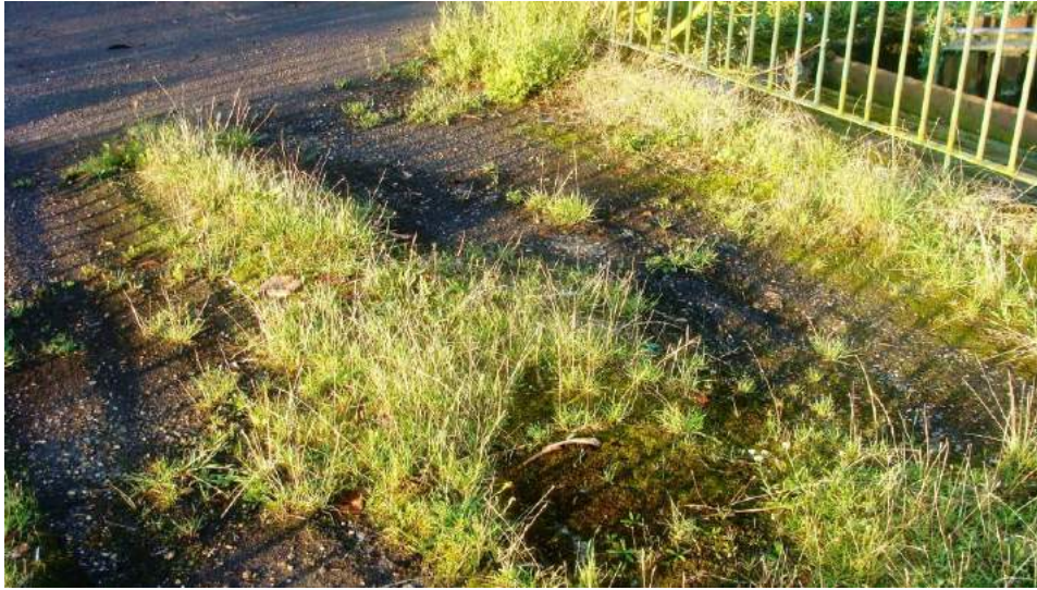
Picture 42. Vegetation on surface to listed bridge Hertford Road in need of removal. It is hoped it remains structurally sound?
