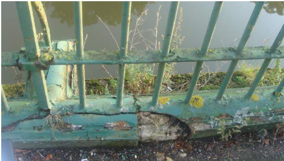
Picture 44. Detail of railings some of which are in need of repair and or repainting. In some areas removal of self set sycamores would be beneficial.
